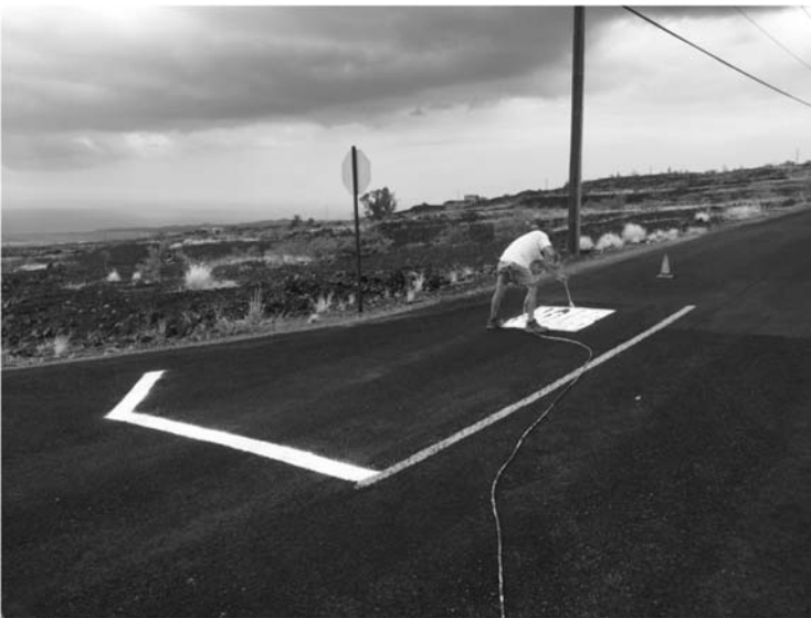
Newly chip sealed intersection is getting stop bars painted.
