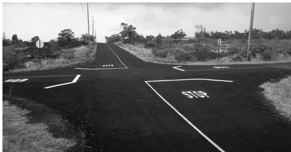
Newly paved and painted intersection
